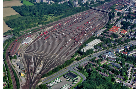
Hagen Shunting Yard, Germany
